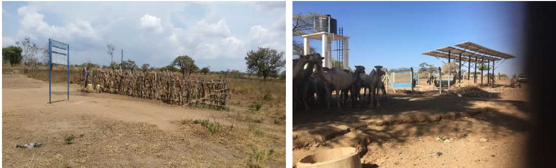
Figure 5: Fenced Borehole and Solar Powered Borehole in Uganda
