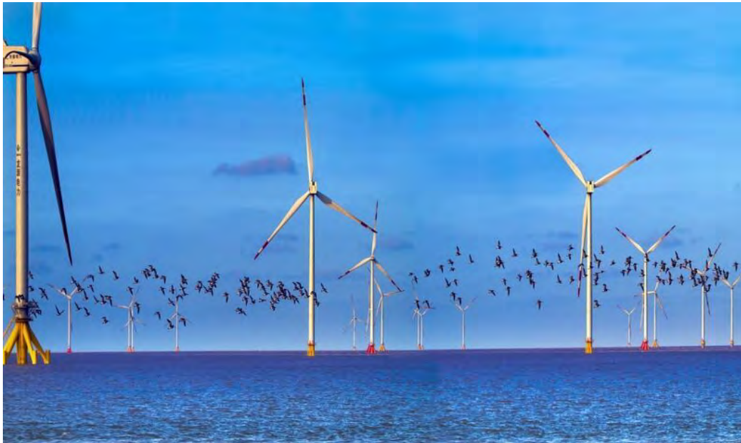
Figure 14 Rudong, Jiangsu offshore wind farm. © Wu Zhenhua
