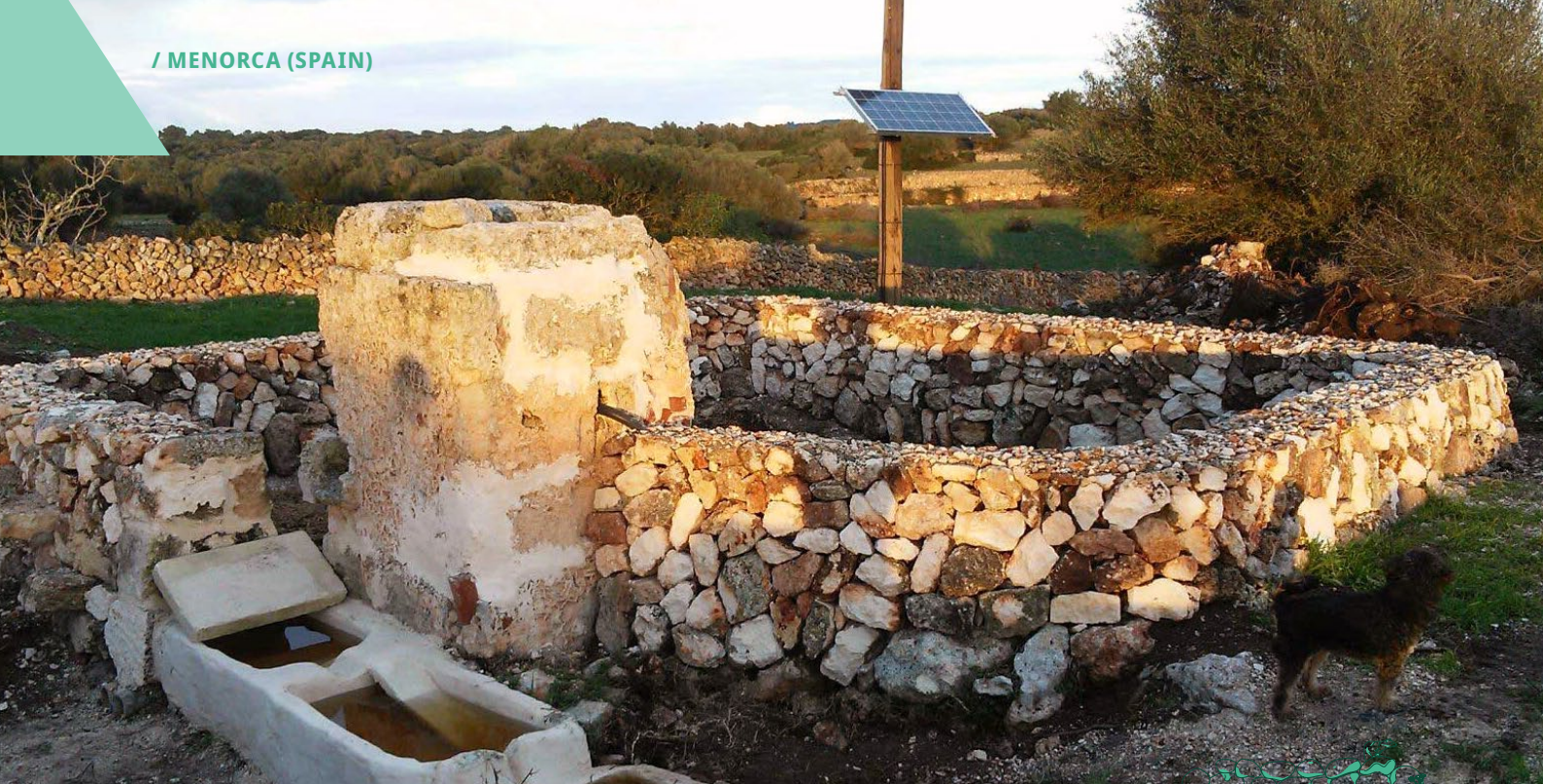
Traditional rainwater harvesting system called aljub . Besides recovering them, GOB builds small water troughs for small wildlife, which are critical in the summer season. © GOB Menorca
