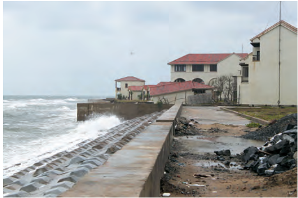
Figure 7: Hoi An beaches are being eroded - Fusion Alya is being sunk to the sea (Source: Axel Neubert)
