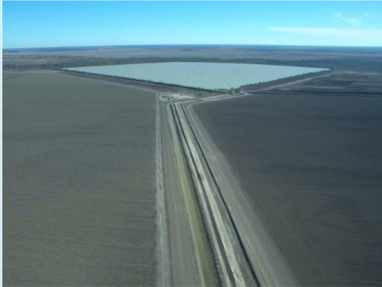
An aerial shot of the Burren Downs dam Water NSW v Barlow [2019] NSWLEC 30
