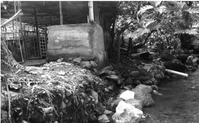
An example of a piggery discharging waste directly into a stream.
