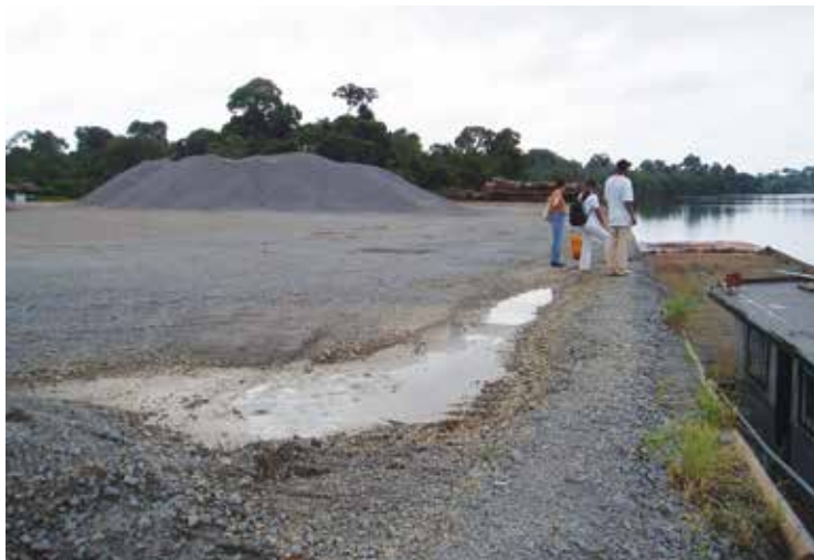
Port expansion area
