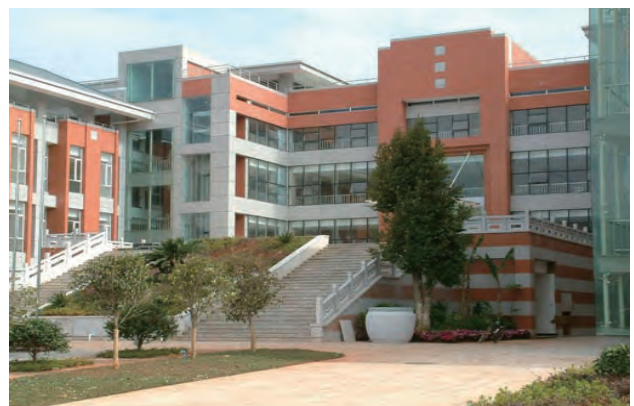
The building of GBOWS 7
