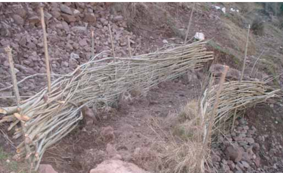
Locally adapted soil stabilization techniques: Abdur Rauf Qureshi, IUCN-AJK 2007
