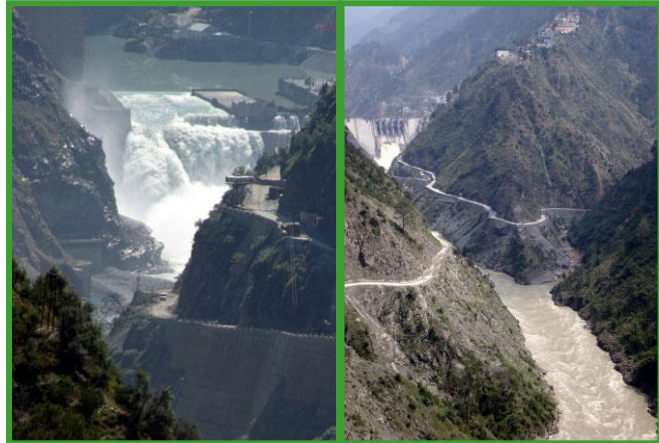
Figures 13 and 14. Baglihar Hydropower Dam in India
