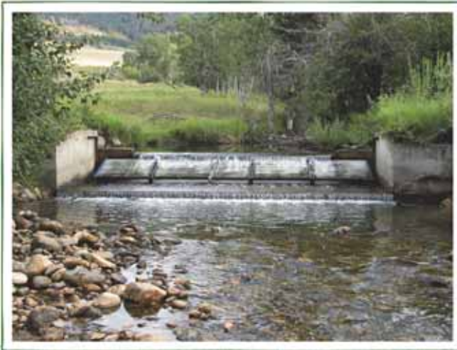
Temporary fish movement barrier on Cherry Creek
