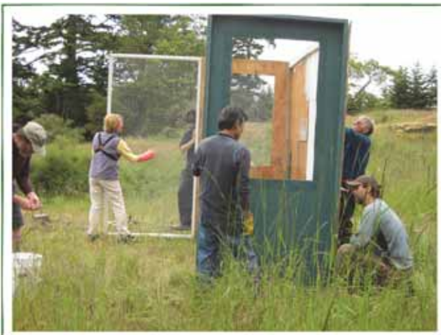
Constructing aviary © Gary Slater
