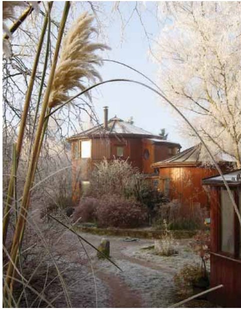
The Findhorn Community Ecovillage in Scotland contains a cluster of "barrel houses" made from recycled whiskey barrels, among other sustainability-minded features.
